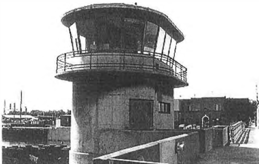
Detail of the control tower. May 2004.
