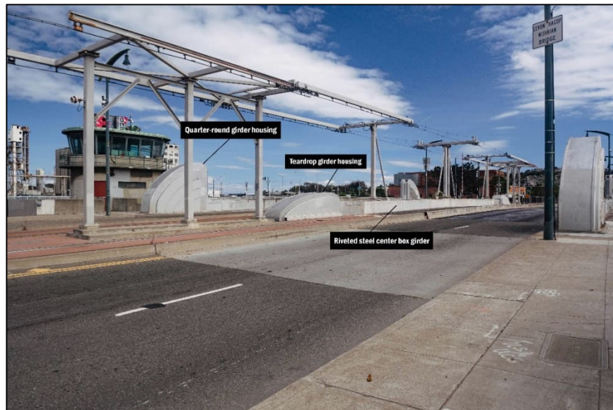
Photograph 1. Above-Deck Character-Defining Features, Including Quarter-Round and Teardrop Girder Housing Units with Art Moderne Styling and Riveted Steel Center Box Girder, Facing Southeast
