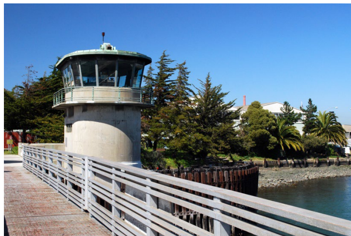
Figure 4 Control Tower and Sidewalk Railing showing Art Moderne Style Applied to Bridge
