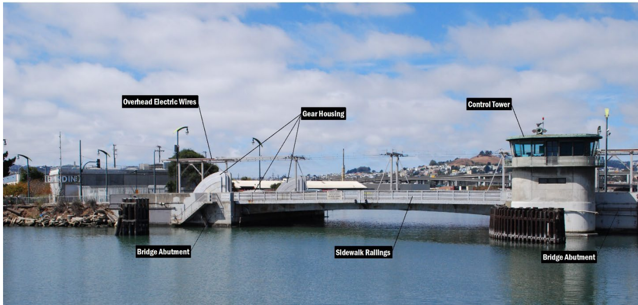
Figure 2 Islais Creek Bridge East Elevation
